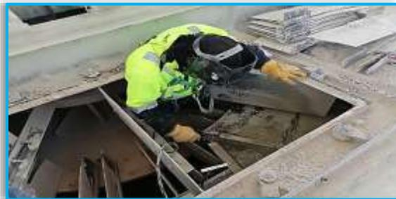
Foto No.15: Soldar placas triangulares
